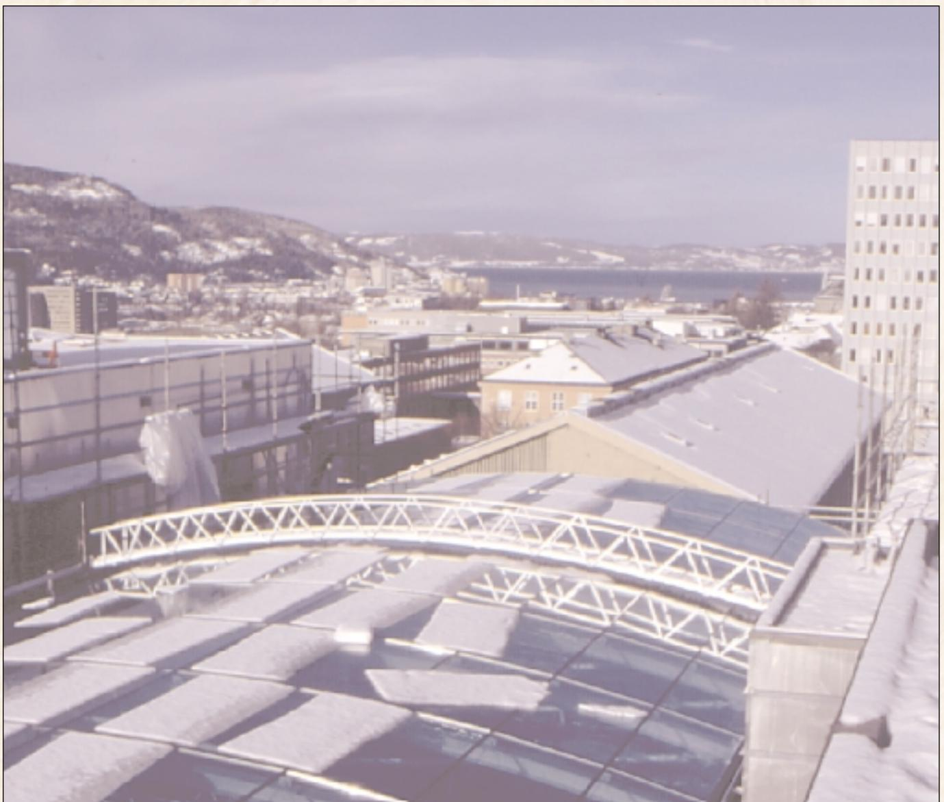
The NorAcon traversing ladder is often used for access to inclined or curved glass roofs as shown in the pictures. It will also provide safe and easy access to vertical facades where the height is limited.
